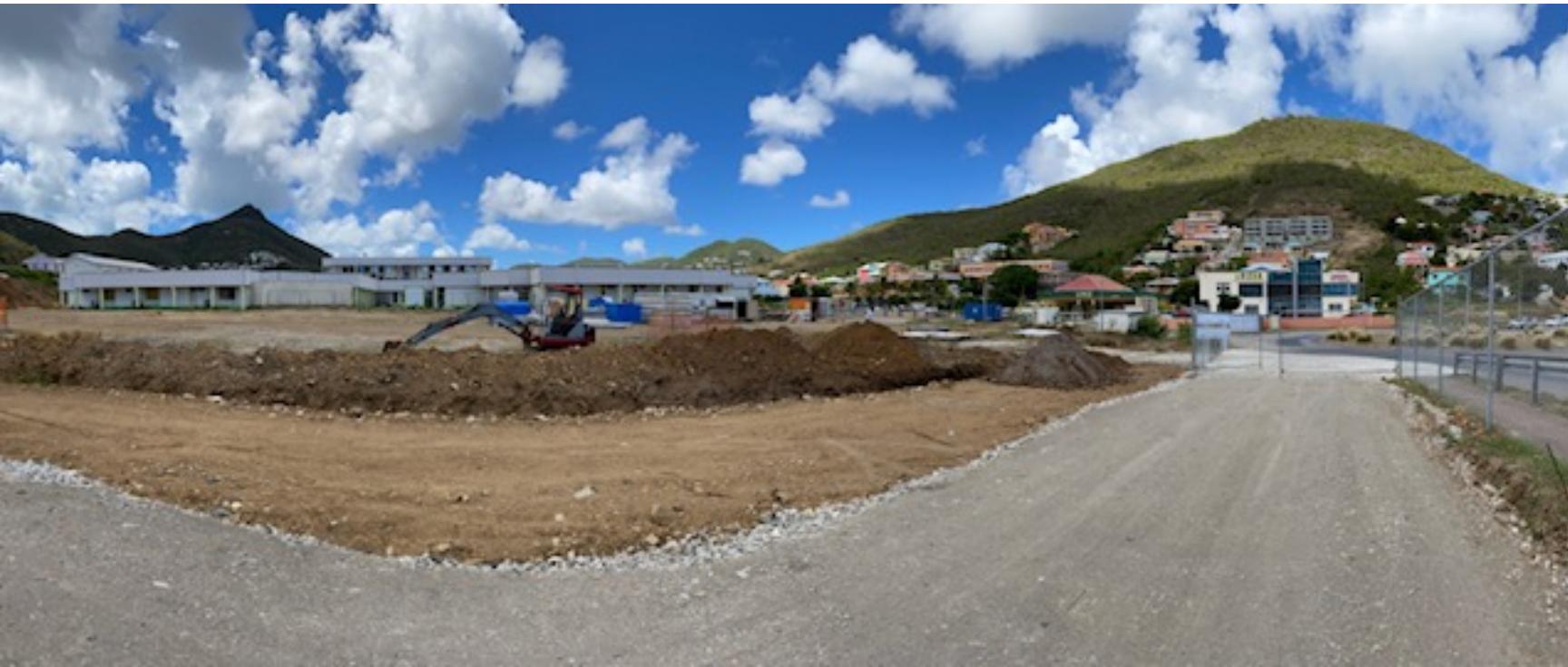
Construction Site Entrance
