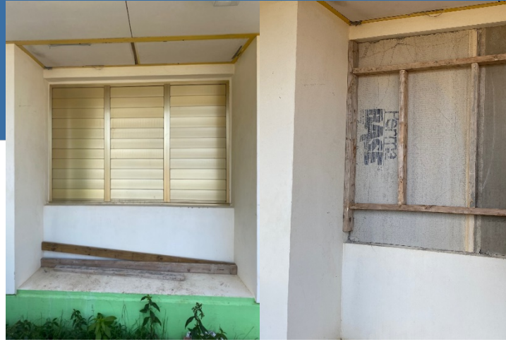
Installing of Acoustic Barrier
